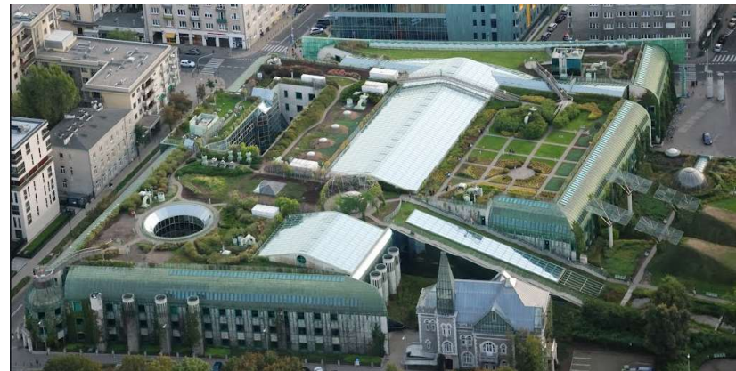
Roof of the University of Warsaw Library
