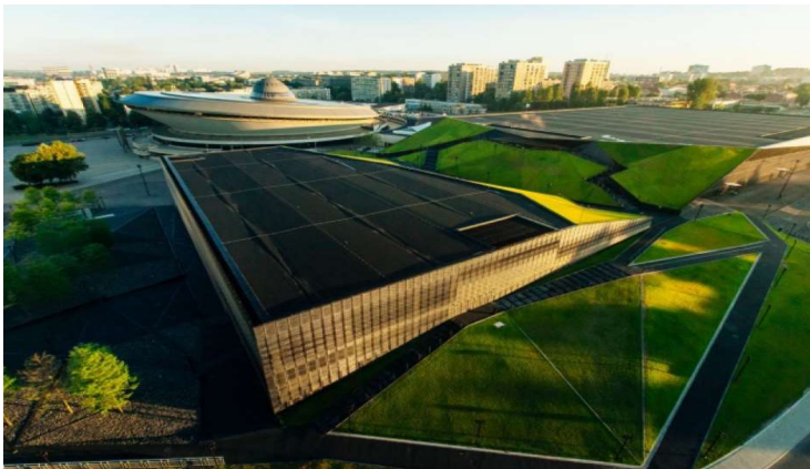
Internacional Congress Centre in Katowice
